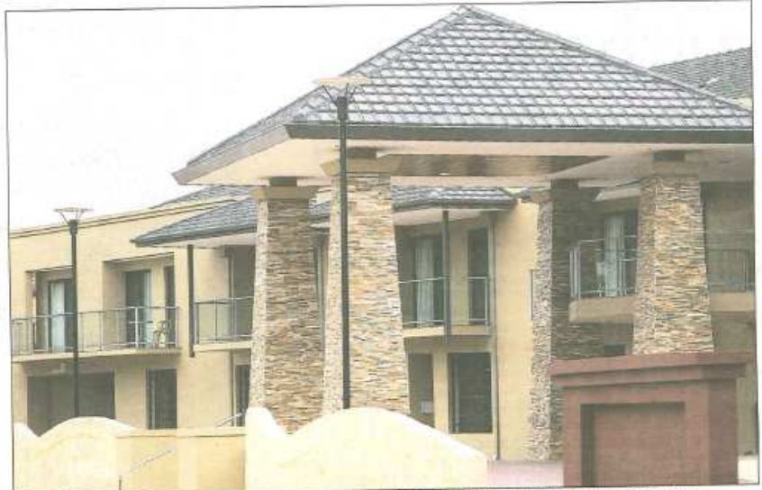
Woodlake Aged Care project won the Master Builders Association's best lifestyle housing for seniors (over $1m).
